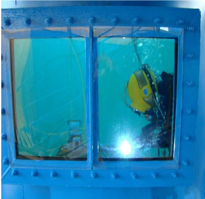
Fig. 1. Student diver practices welding underwater. Adapted from [5].
