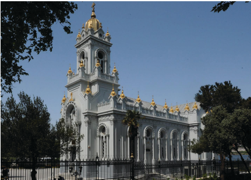
Figure 13. St Stephan church after restoration in 2018. Photographer Tsvetan Tomchev.
