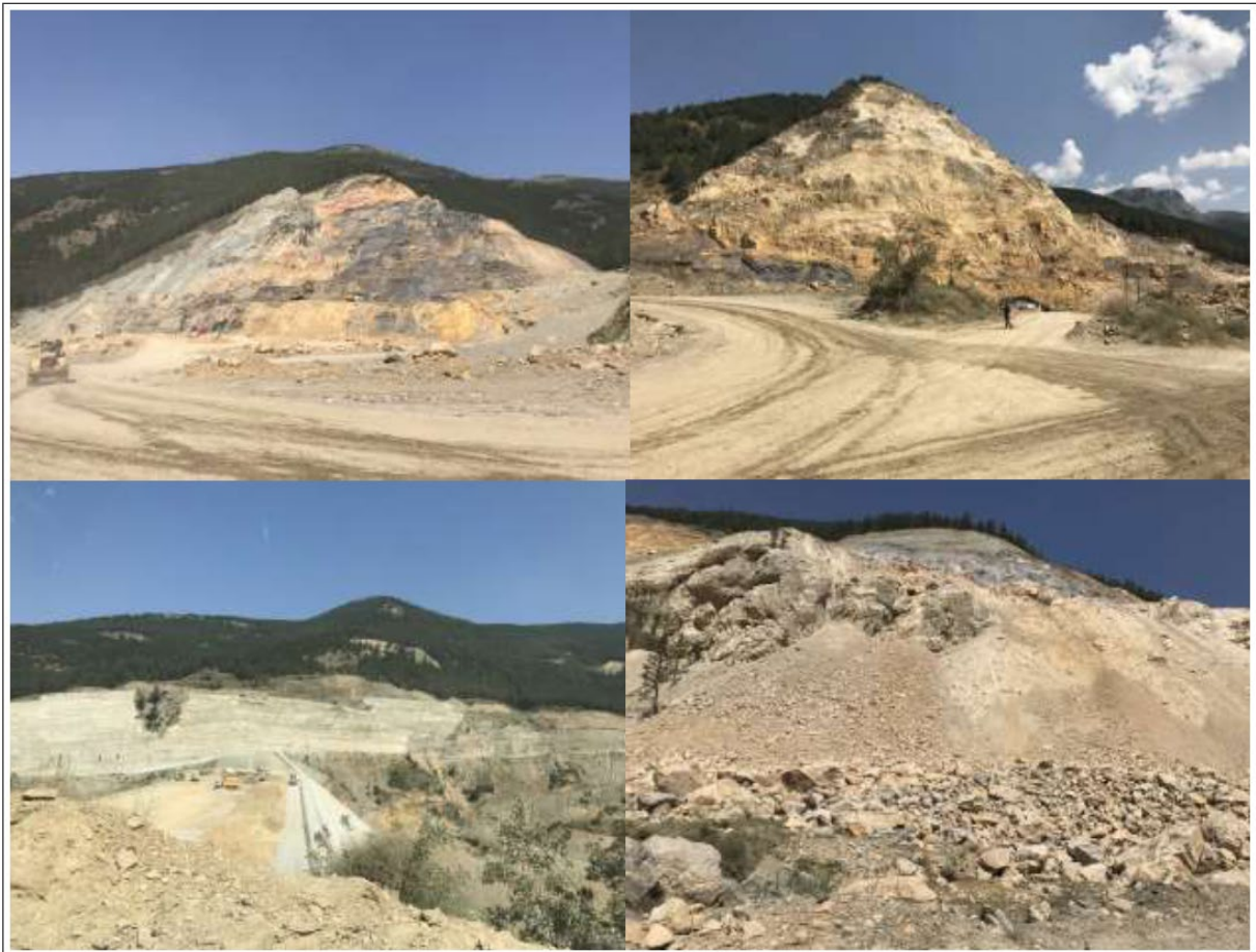
Figure 13 - Blast locations conducted for the embankment of Çay Dam.
