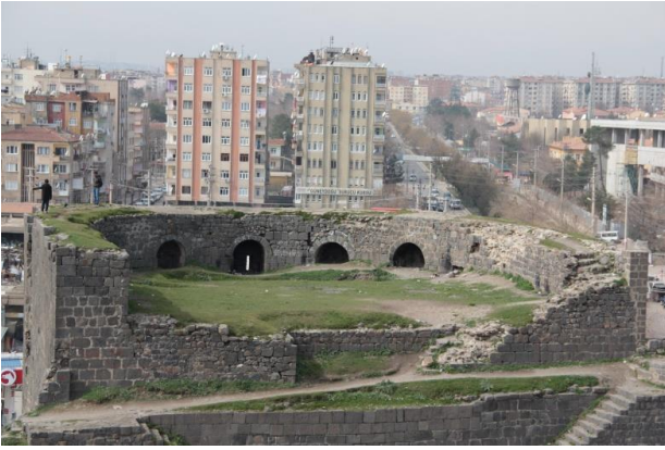
Figure 7. The photographic view of the top of Tower 20
