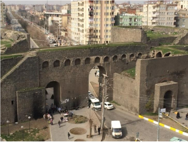
Figure 10. A photographic view of porticos on the Urfa Gate
