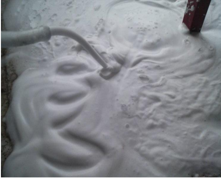
Fig. 5. Making of foam using foam generator
