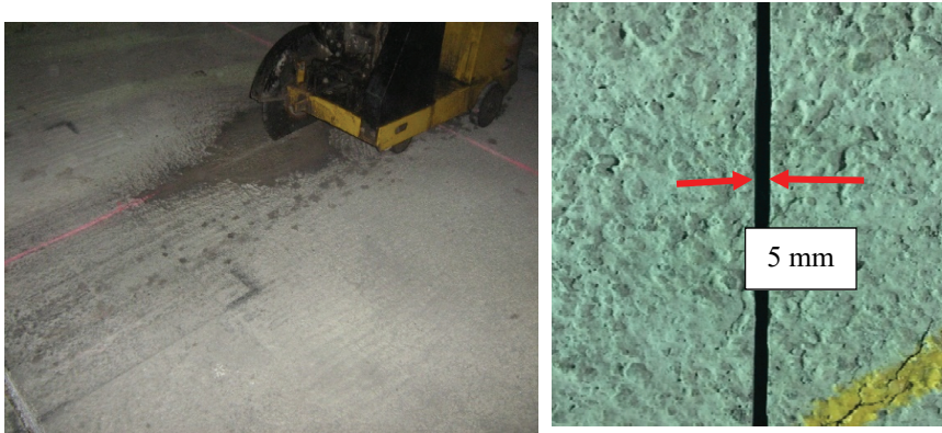
Figure 6 - Saw-cut contraction joint and joint openings
