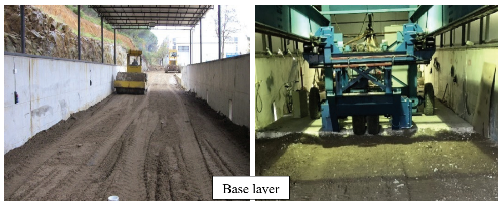
Figure 5 - The base layer beneath the concrete pavement
