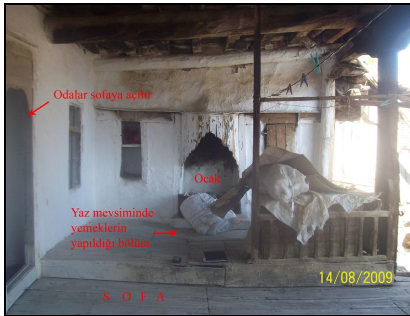
Foto 3. Eski tip konutlarda dış sofadaki mutfak işlevi gören bölüm. (Photo 3. The section that was used as a kitchen in the exterior hall of old-style houses)
