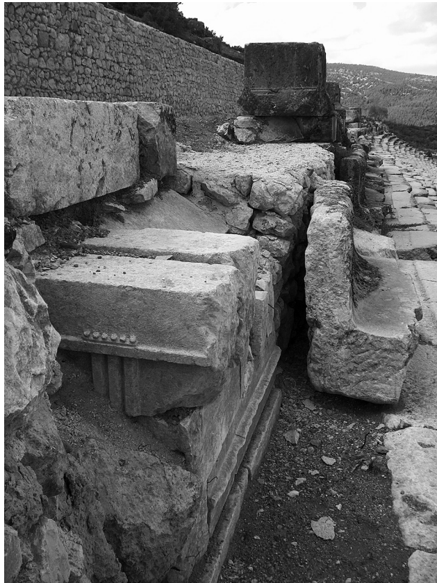
Fig. 16 Spolien material re-employed in the foundations of the Portico bases on the west seating rows of the stadium.
