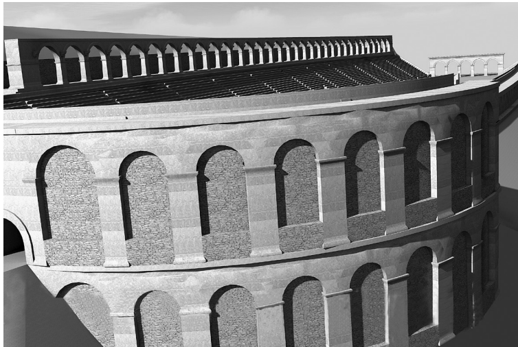
Fig. 10 Sphenoidal vaulted arch support for south-eastern two-storey retaining wall (Architects I. Akgül – N. Gürlesin – M. Sayan – N. Kocaman).
