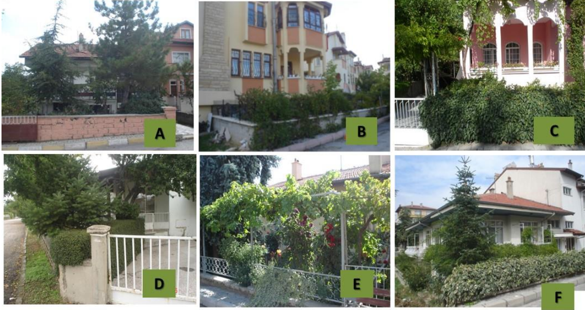
Figure 5. Front views of some detached family house garden's walls (walls of- A : plastered briquette; B-D : Concrete and plant on it; E : Stone-metal plant on it; F : Concrete-metal plant on it).
