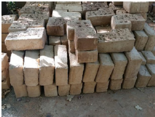
Figures 3 & 4. On-site stabilised earth block production of a demonstration building project constructed in a residential area of Bloemfontein, South Africa (2016)
