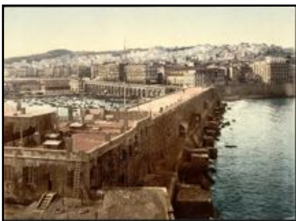
Figure 2. View of the Kasbah of Algiers
