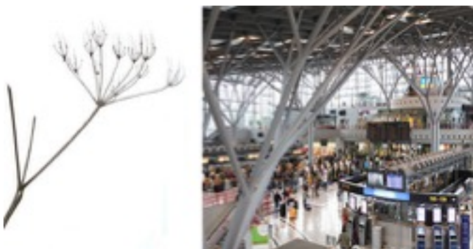
Figure 12. Stuttgart Airport Passenger Terminal by Von Gerkan and Partners (Von Gerkan, 2007). This roof was designed by directly adopting the branching theory of Frei Otto.
