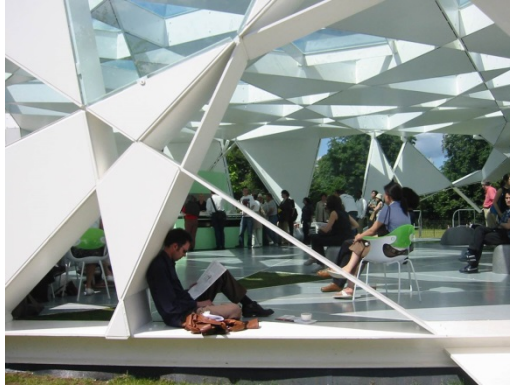
Figure 5. Toyo Ito, Serpentine Gallery Pavilion, London, United Kingdom, 2002
