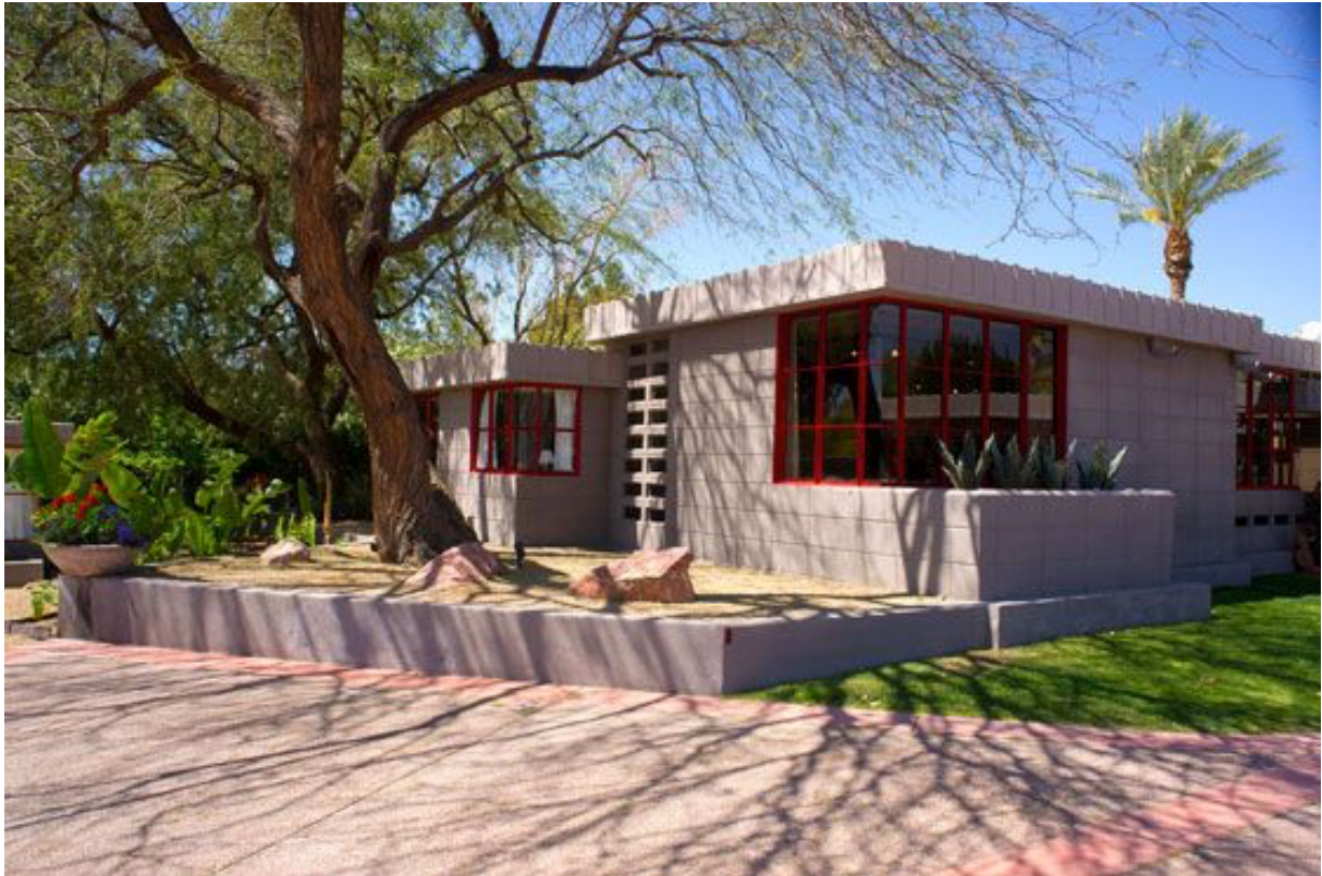
Figure 10: In Benjamin Adelman House (1951), two different kinds of openings are located side by side. Both are fixed windows. The differences are the sizes and locations of the openings. Photo: Shuttermike Photography, 2012.
