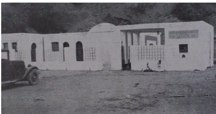
Figure 3: Hammam Melouane - Restoring of the Marabout pool of Sidi-Slimane
