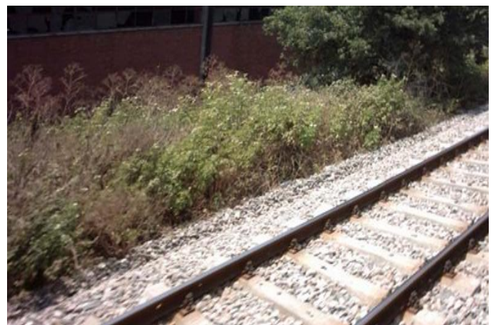
Fig. 3. Vegetation on and around the railroad in İzmit.
