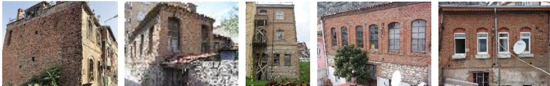
Figure 42. Examples of traditional Eğırdır houses which has stone masonry ground floors and brick masonry upper floors.
