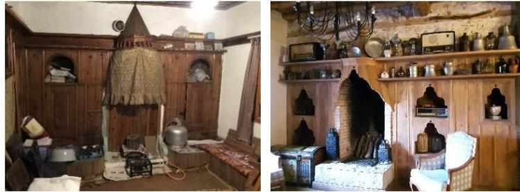
Figure 22. Example of ovens with timber hood “yaşmak” at the traditional Eğirdir houses
