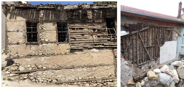
Figure 39. Using stone and timber framed system together in traditional Eğirdir houses
