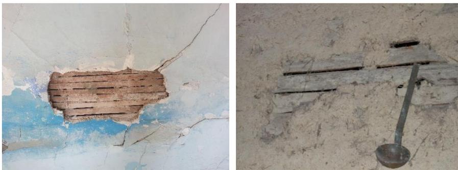
Figure 43. Examples of timber lathed “bağdadi” plaster at traditional Eğırdır houses
