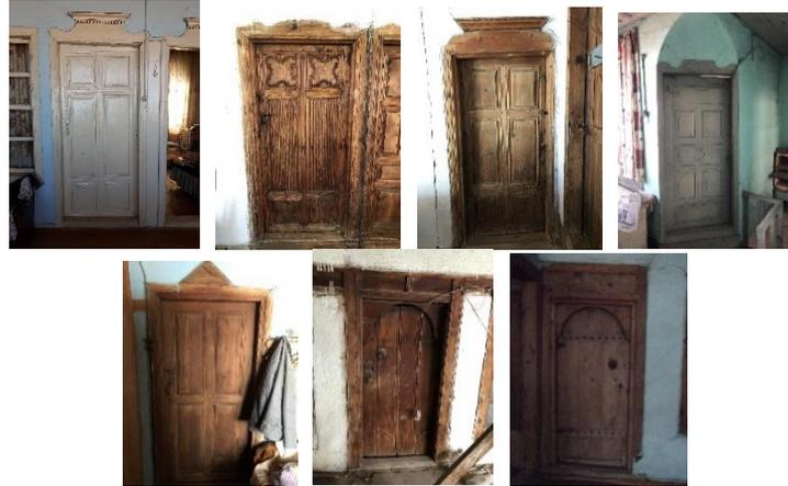
Figure 16. Example of interior single winged doors which have profiled or arched pediment in the traditional Eğirdir houses
