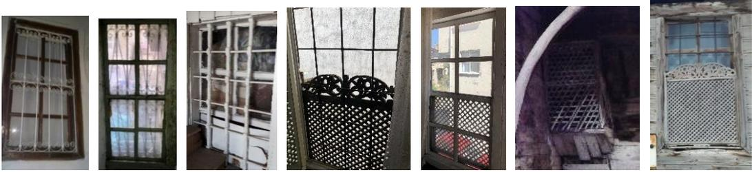
Figure 20. Examples of metal and timber railings on windows of traditional Eğirdir houses
