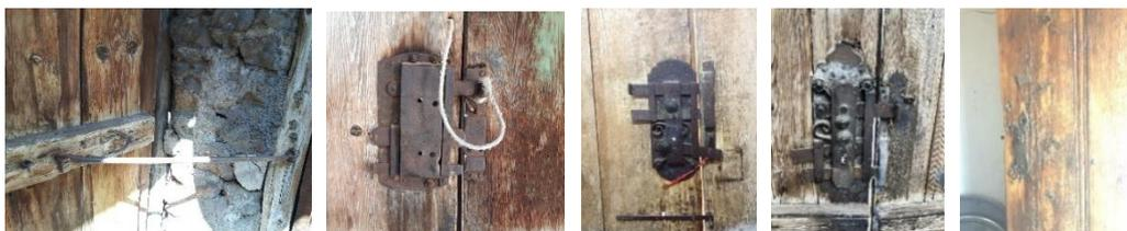
Figure 19 Examples of locking mechanisms of the exterior doors of traditional Eğirdir houses
