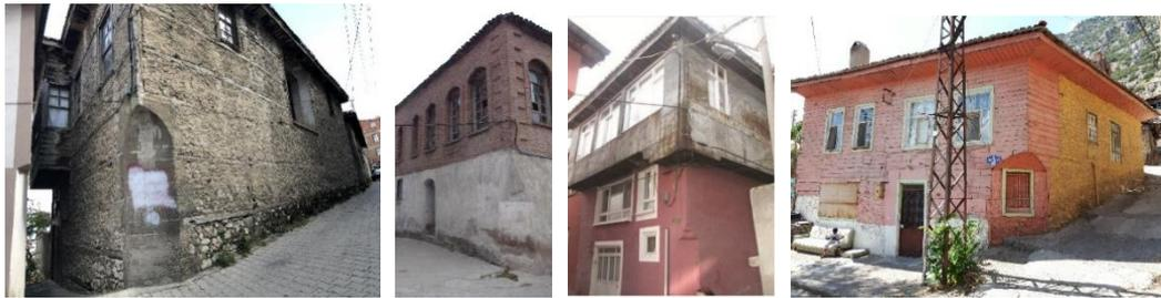
Figure 45. Example of chamfered corners at Traditional Eğırdir Houses
