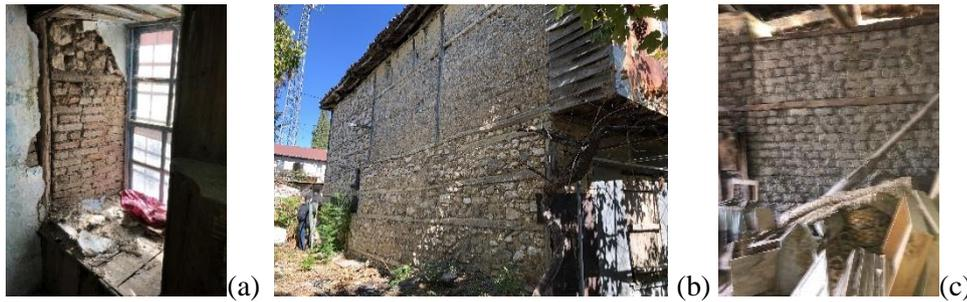
Figure 41. Wall fillings at traditional Eğırdır houses (a), brick filling (b), (c) adobe filling
