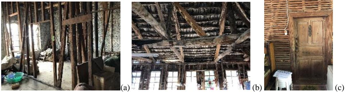
Figure 40. Traditional Eğırdır houses (a),(b) examples of timber framed system, (c) timber lathed “bağdadi”
