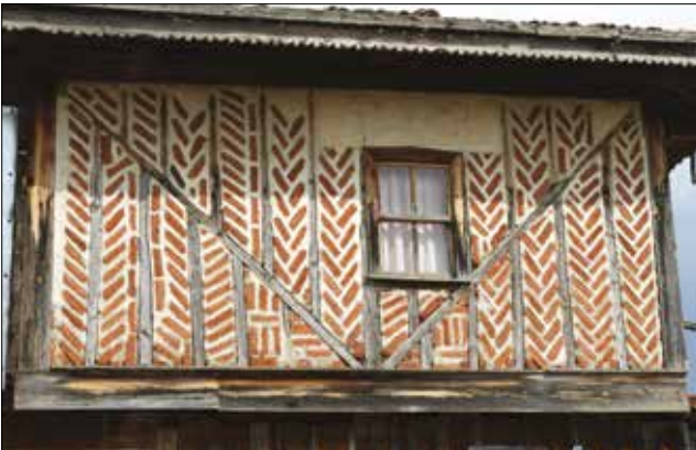
Fotoğraf 50. Ahşap çatkılı ve tuğla dolgulu "camlı ev" (oda), Terzi Ahmet Köyü / Timber framed and brick infilled "camlı ev" (the room with glass), Terzi Ahmet Village, 2018.
