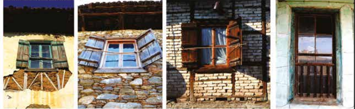
Foto. 8-15: Pencere ve kepenkler Photo. 8-15: Windows and shutters
