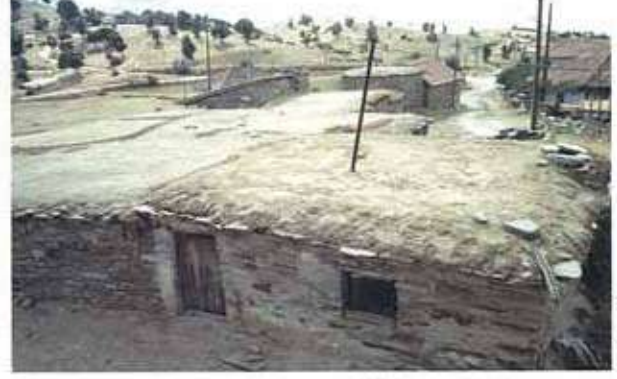
Res. 52. Ali Maden evi (env. no: L21C011.048), Aşağı Mahalle, Karaköy.
