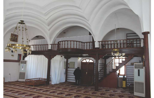
Fotoğraf 22 - Şebinkarahisar Tamzara Mahallesi Camisi mahfil ve kubbe destekleri / The gathering place of Şebinkarahisar Tamzara Neighborhood Mosque and its dome's supports
