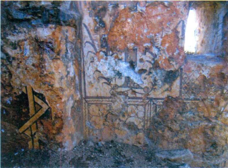
Fig.12 - The detail from "eight-cornered star" motive and the south wall.
