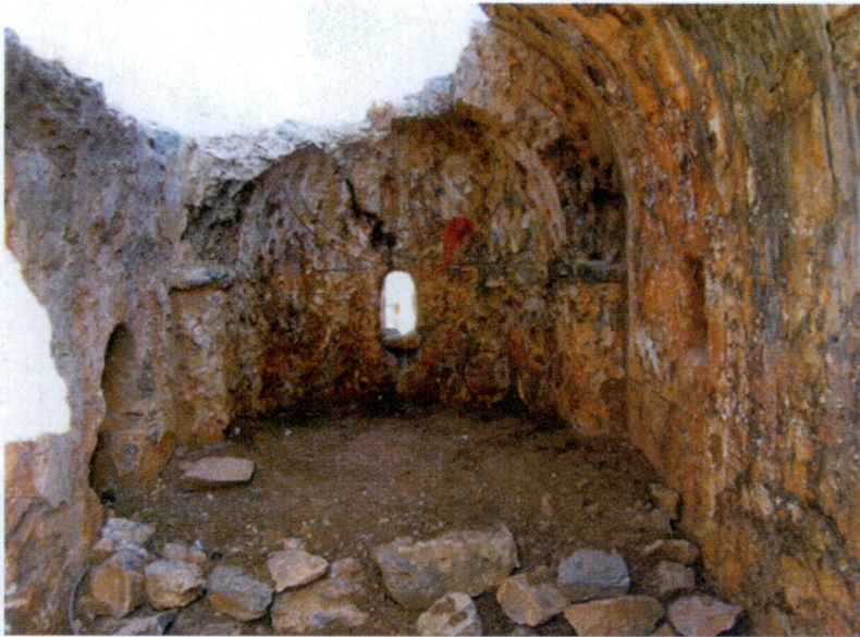
Fig.2 - Internal view (from west to east)
