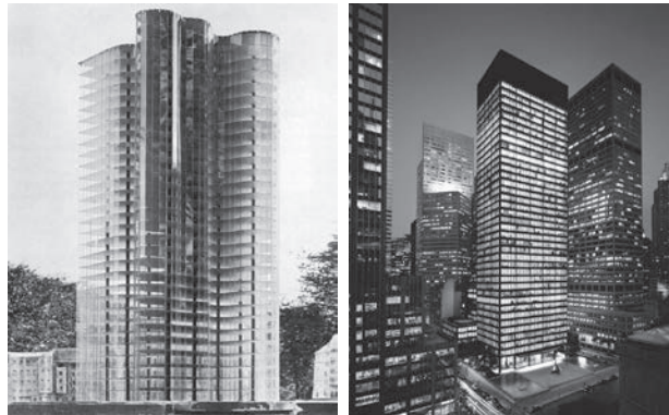
Figure 2. "Non-ornamental" buildings of Modern architecture Industrial materials, forms and machine aesthetics Left: Model for a modern glass skyscraper, Mies van der Rohe, 1922 [14] Right: Seagram Building, Mies van der Rohe, Philip Johnson, New York, USA, 1958 [15]
