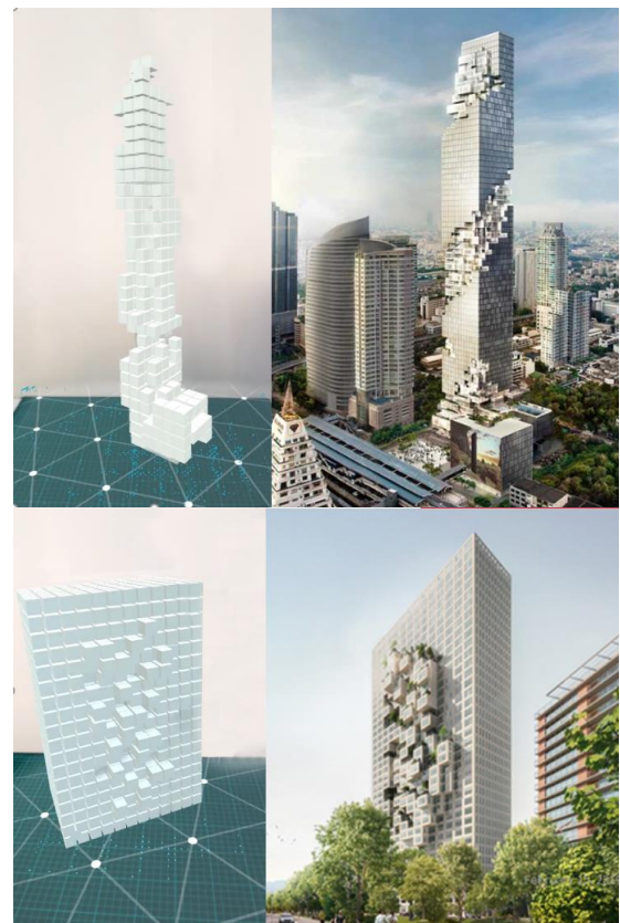
Figure 13: Example studies for two different masses using virtual bricks method (Url-5, Url-6).
