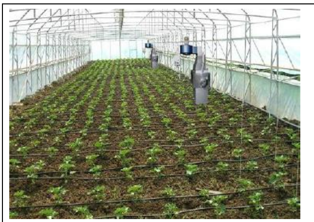
Figure 3. Biogas used for heating in the greenhouses [2].
