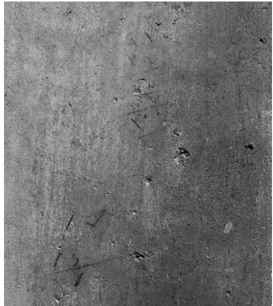
FIG. 9 Records written in Ottoman Turkish on the front face of the left side of the door frame of the entrance to the Yenikapı Hamamı (Bathhouse).
