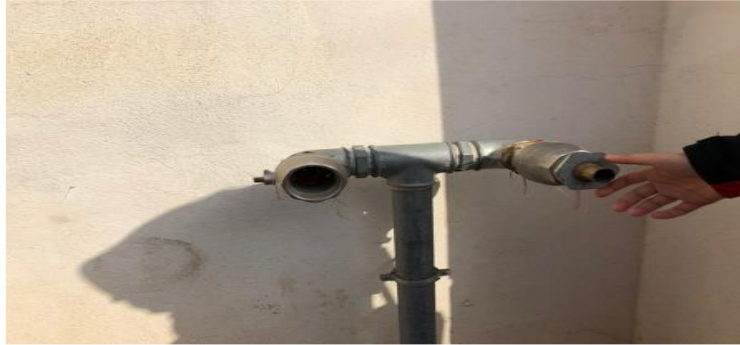
Figure 4. Keeping Obstacles on Emergency Exit Roads
