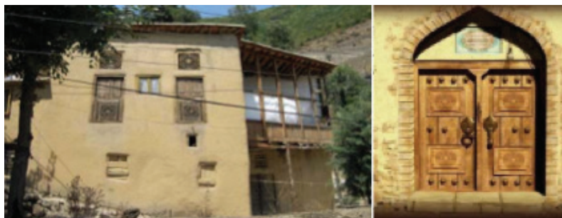
F. 8: a. Aesthetic elements in Masouleh (Kakouei et al, “Masouleh: A City; A History,” 2846), b. Aesthetic elements in Masouleh (Imani Emadi, et al, “Sustainable Architecture Analyses of Stepped Village, Case study: Masouleh, Iran,” 154).
