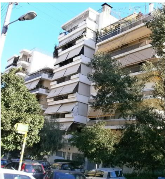
Fig. 1. The block of flats (building in the middle) where the apartment of the case study belongs
