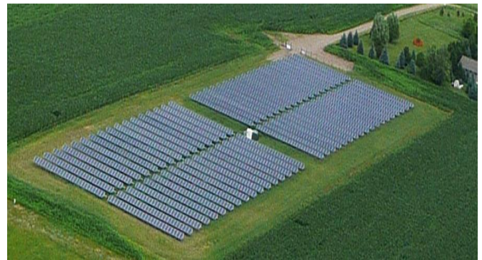
Fig. 1. Appearance of a PV system with a power of 1 MW consisting of 4,000 modules of 250 W each.
