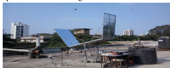
Figure 3. Hybrid PV/T solar water system with measuring instruments
