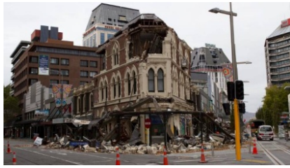
New Zealand, Christchurch (Stuff, 2020) 22 Feb. 2011/ 6,3 Mw
