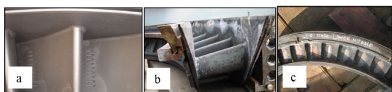
Figure 11. Visual inspection of 1st stage turbine nozzle (a) before operated (b) after operated by HSD taken on Major Overhaul (c) after operated with B5 for 1 month
