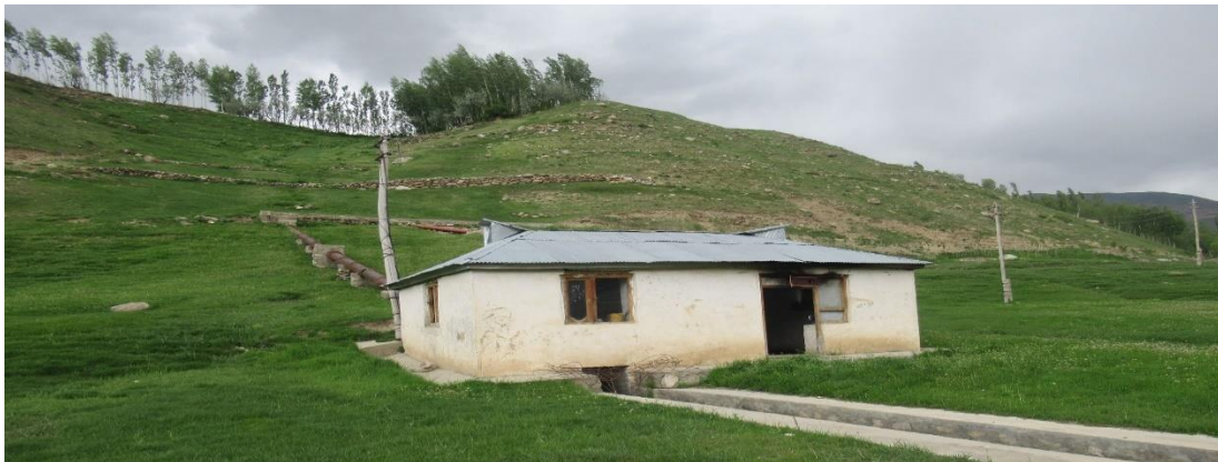
Picture 1: A view of Micro-hydro Power Plant- Badakhshan Province –Afghanistan
