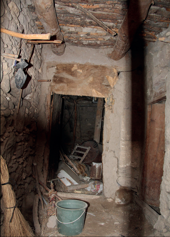
Fotoğraf 62: Zemin Kat Tavan ve Döşeme / Ground Floor Ceiling and Flooring
