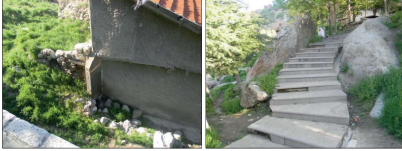
Figure 9: Lower Castle gate, jamb pieces and castle exit stairs (Köker, 2020)
