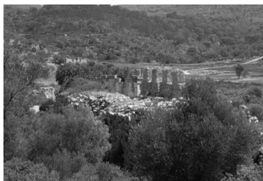
Fig. 6. Parapet and merlons that retain traces of insitu Seljuk paintwork
