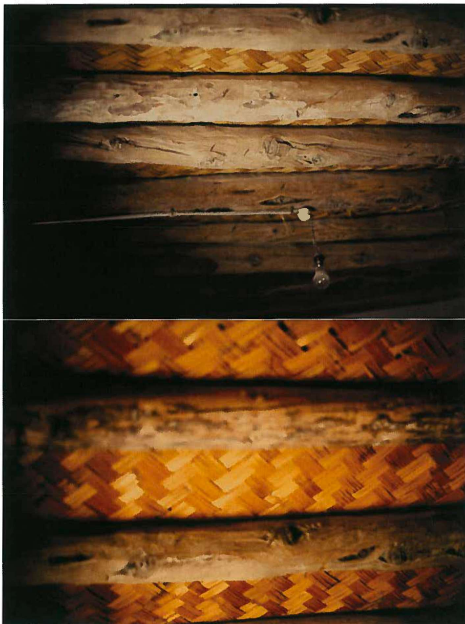
Fig 4: Roof matting using B. maritimus stems. In the Konya Basin today, village women flatten and weave the stems of sea club-rush into matting that is used to cover the ceiling in some rooms (Adakale nearby Hotamış Sazlığı).
