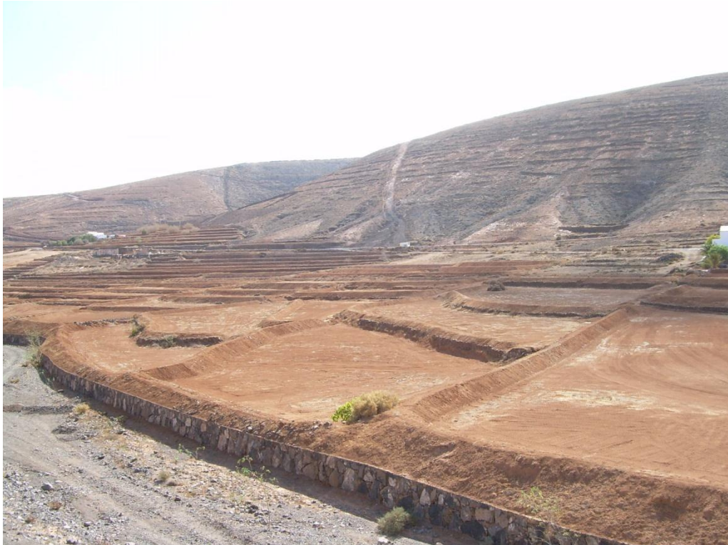
Figure 3. Earth dams, to intercept surface water, called Gavias in Fuerteventura Island, Canaries, Spain (Santamarta, Cerezal 2007).
