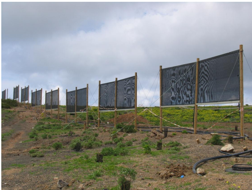
Figure 2. Fog collectors in Lanzarote Island, Canary Islands, Spain (Santamarta Cerezal, 2008).
