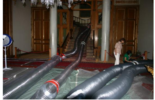
Şekil 6. Koridor ve ikinci kata giden gaz boruları Figure 6. Gas pipes going along the corridor and to the second floor
