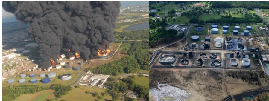
Figure 1. Photos of the accident site (Doğan, Scarabella and Akman, 2020).
