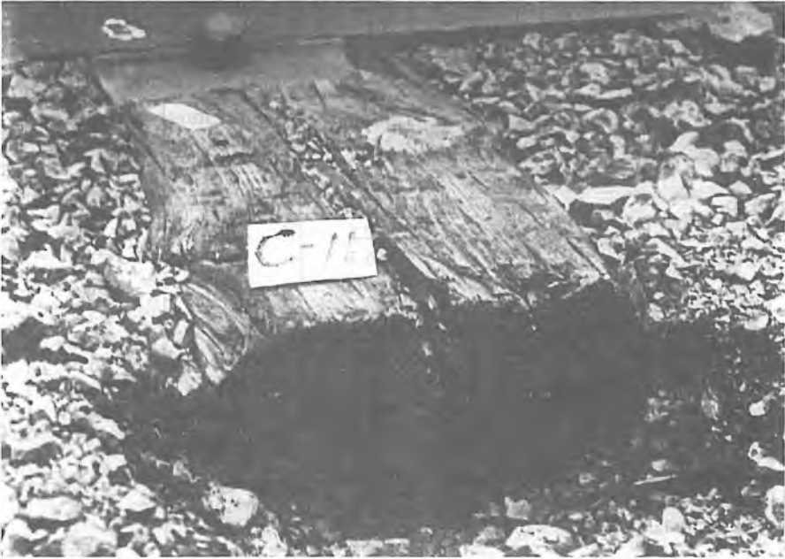
Figure 1: Ties examined in North-Bay. A typical laminated tie (above) and a control tie
