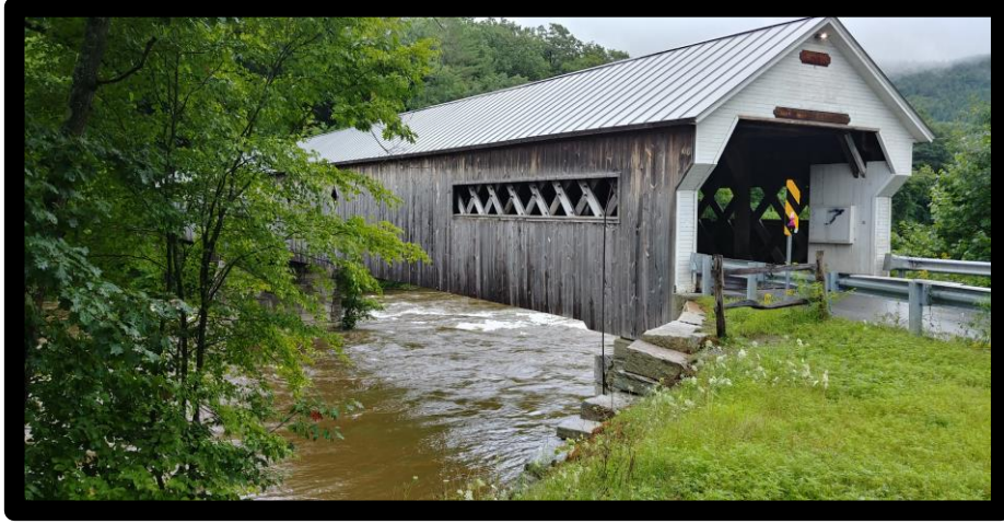
Fotoğraf 7. West Dummerston Covered Bridge, Vermont.
