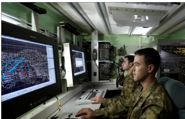
Fig. 4. Shelter Mounted C2 System
