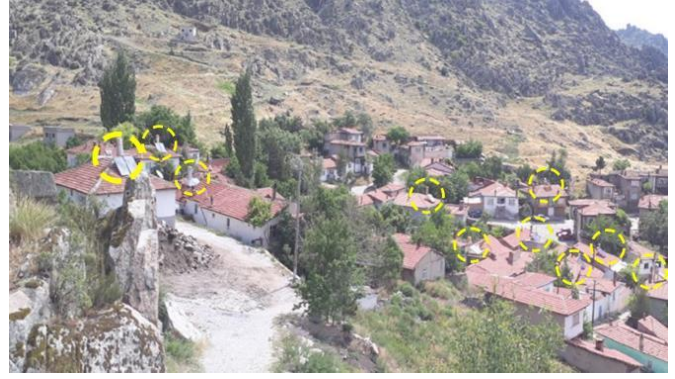
Figure 5: Sivrihisar "Rooftop" Solar Heating Systems
