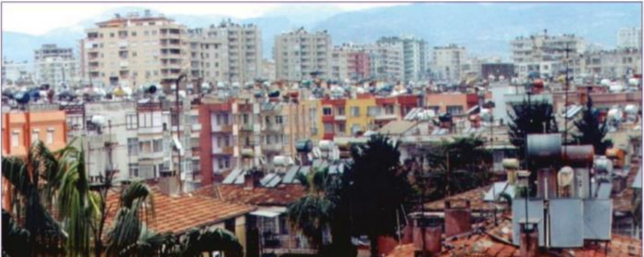
Figure 2. Solar Heating Systems in Mersin Context (Sakinç and Sözen, 2009)
