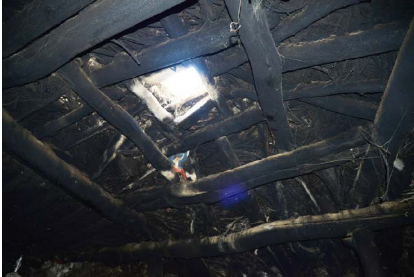
Figure 12 - Inside of the dome of the Tandoori house.
