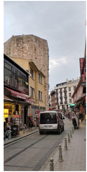
Figure 9: The Nevbethane, one of the two octagonal towers of the Topkapı Palace's outer wall. Photograph: Ezgi Dikici, December 2019.
