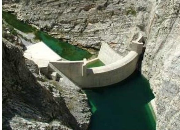
Şekil 1. Beton gövdeli Berke barajı (Figure 1. Berke dam is concrete-bodied)
