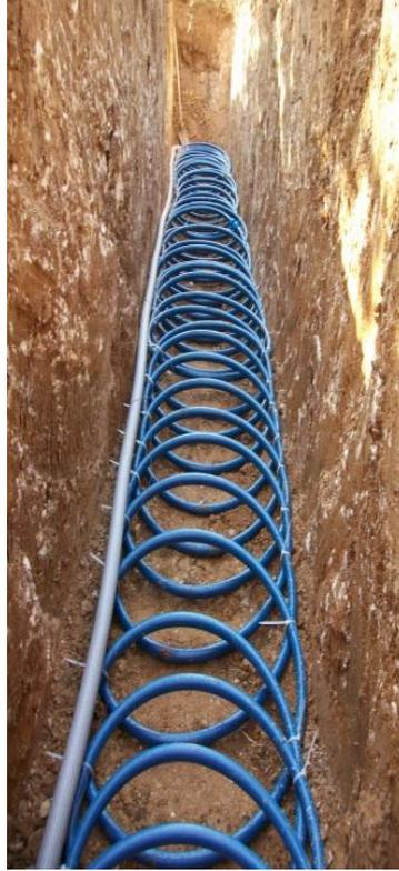
Figure 1. The view of slinky pipes [16]
