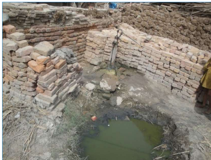
Fig. 6. Poor drainage causing groundwater contamination in study area
